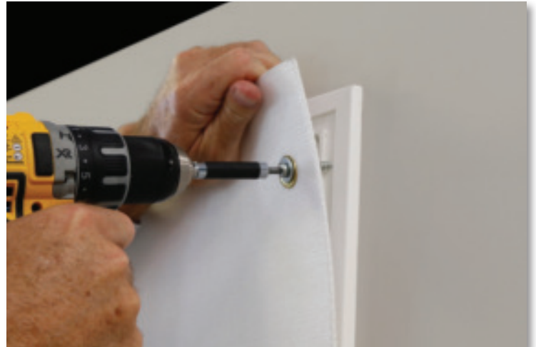
Align hurricane panel. Use Muhler screw to attach panel. By placing hurricane panel on the door, the door can function as an egress method.
