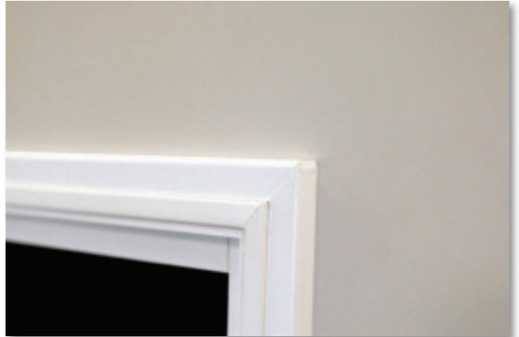
Welded corners. Miter cut stops eliminate screws and, more importantly, screw hole plugs.
