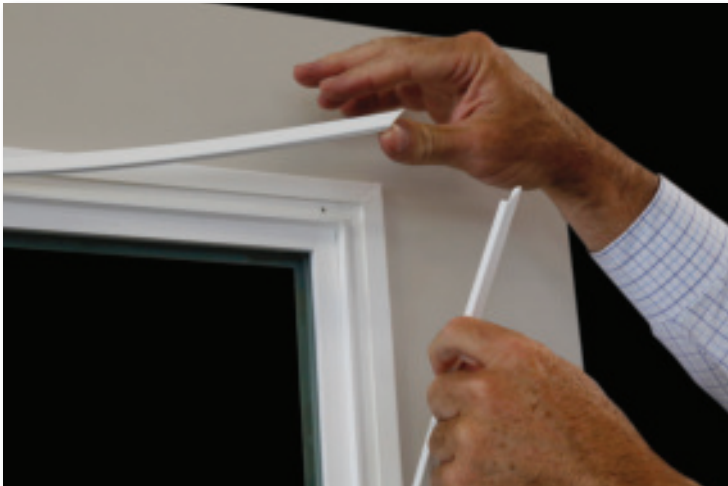
When using non-impact glass and hurricane panels, remove cover caps.
